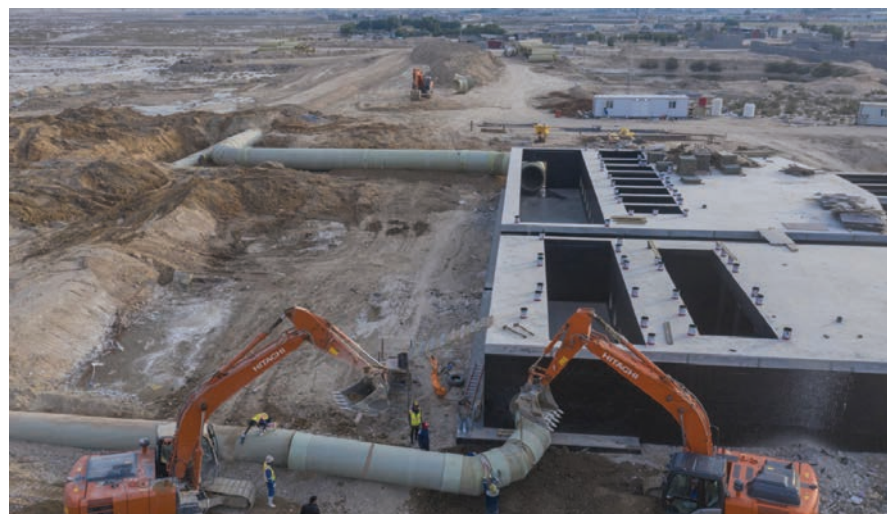
Al-Askari/Zubeir PS6 (Sewer (860 l/sec) and Stormwater (9,800 l/sec))
