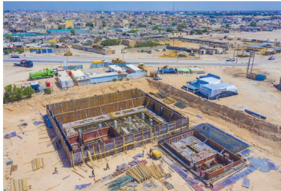
Al-Mribad/Zubeir PS1 (Sewer (2,390 l/sec) and Stormwater (7,110 l/sec))
