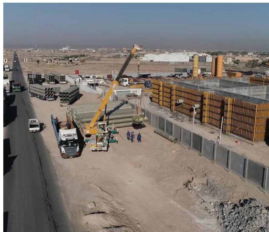
Al-Askari/Zubeir PS6 (Sewer (860 l/sec) and Stormwater (9,800 l/sec))
